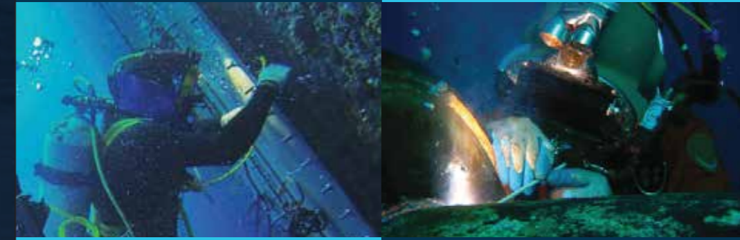
Underwater Blanking Seachest
